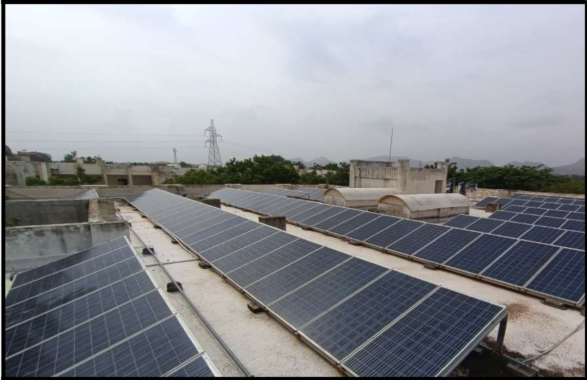
SOLAR PANELS OF 45 KW ON-GRID i.e. NET METERING
