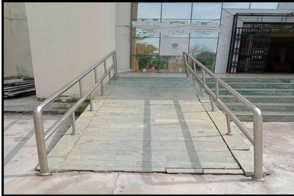
RAMPS WITH RAILINGS & WHEEL CHAIR
